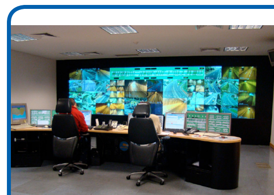
Traffic management, SCUT toll, Control of 30 tunnels in the ER-1 express road and Control Centre in Funchal (Madeira-Portugal, VIALITORAL).
