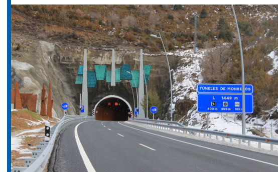
Traffic management, control of 6 tunnels in A23 and the Monrepós management centre (Huesca-Spain, Ministry of Public Works).
